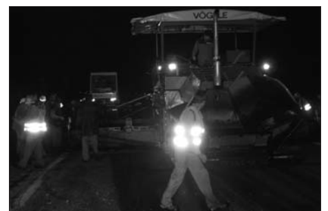
Reflective vests greatly improve workers' visibility
