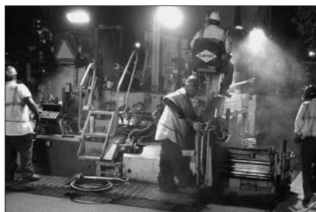
Night-time work area is limited by the range of lighting
