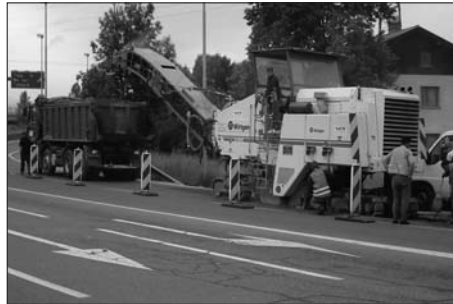
During road closures movement of workers and machines is restricted
